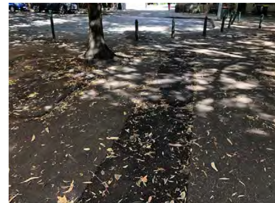
Plate 4: Image showing new trenching below Tree 3. P.Vezgoff
